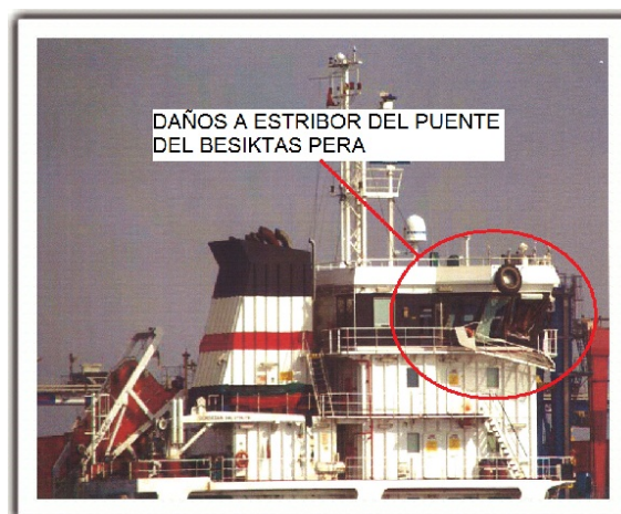
Figure 2. Damage to BESIKTAS PERA
