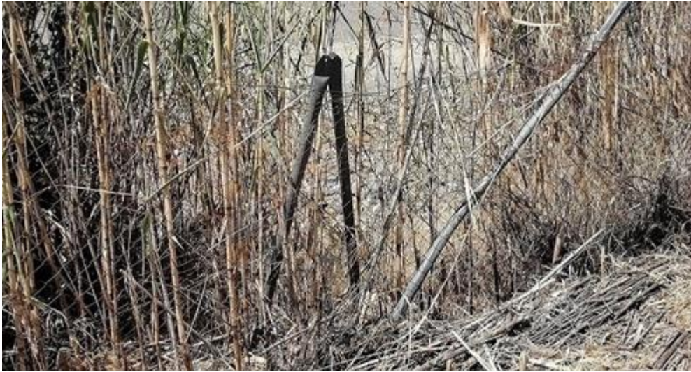
Figure 1. Damage to metal fence
