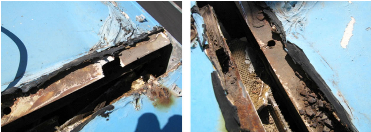
Figure 3. Close-ups of the cabin's top frame
