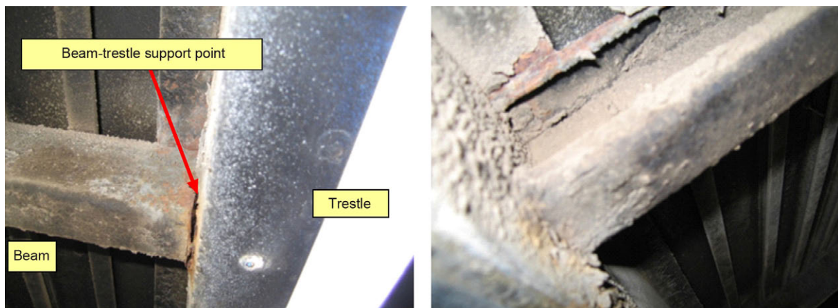
Figure 5. Close-ups of the crossbeam-trestle union
